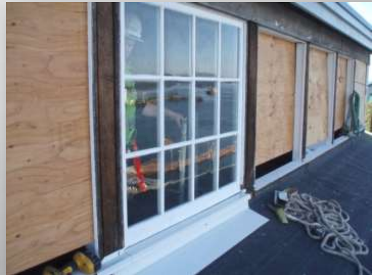
Reinstallation of original windows
