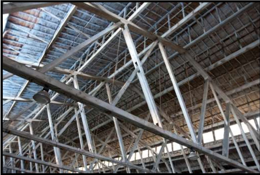
Howe Bridge Truss Construction
