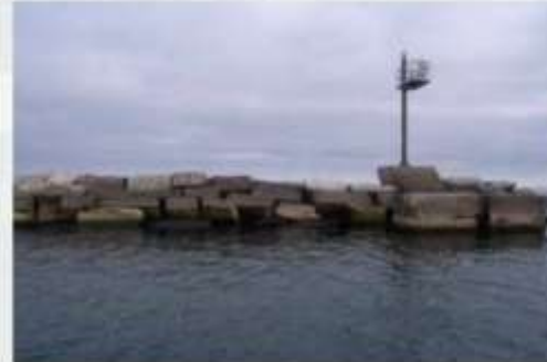
Rubble Mound/Laid-Up Stone Structures
