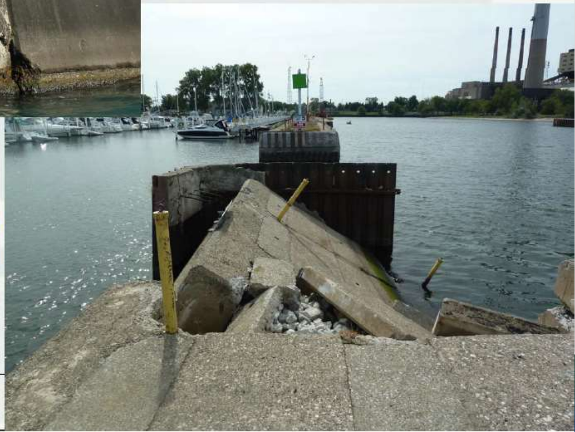
Michigan City, IN East Pier Failure
