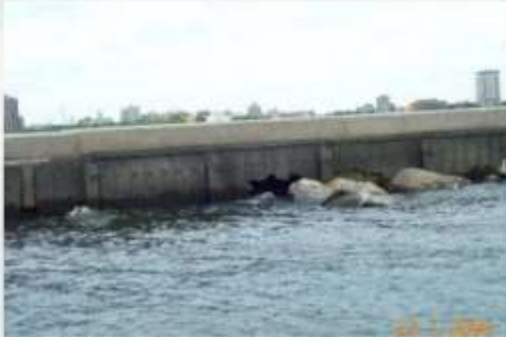
Steel Sheet Pile Structures
