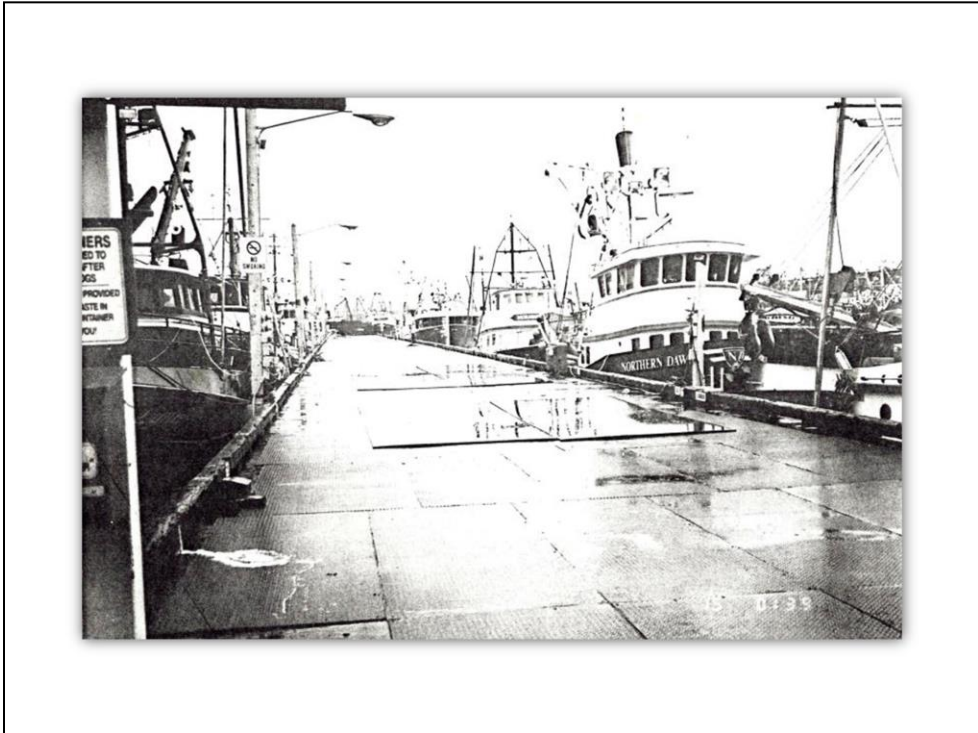
Steel sheets laid atop unsound planks on Dock 5. Vehicles prohibited - hand cards only.
