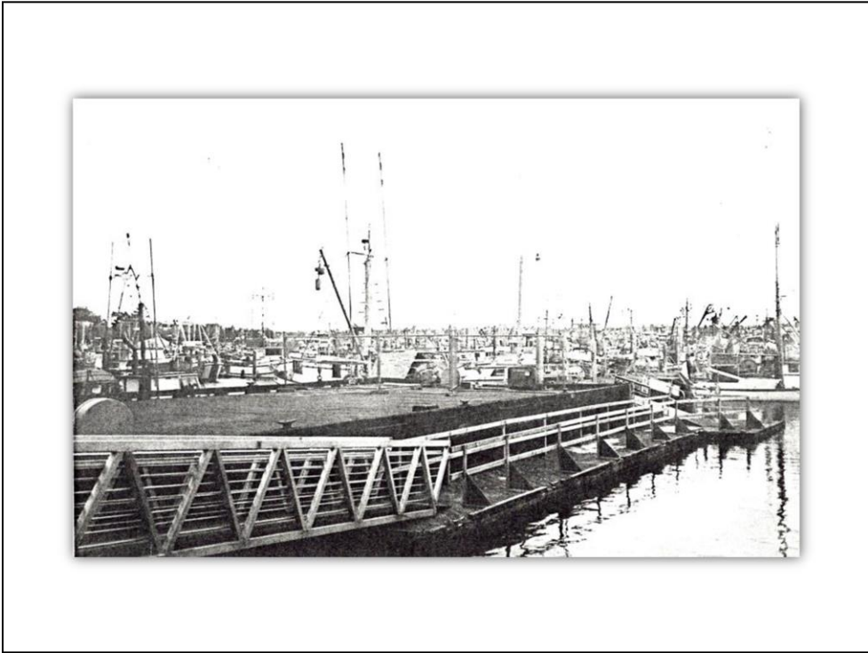
Fishermen's temporary access around condemned infrastructure
