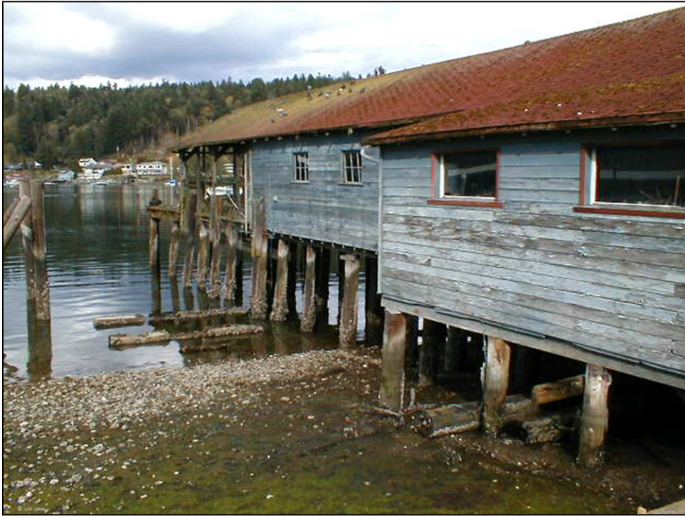
Phase II to restore the netshed is underway.
