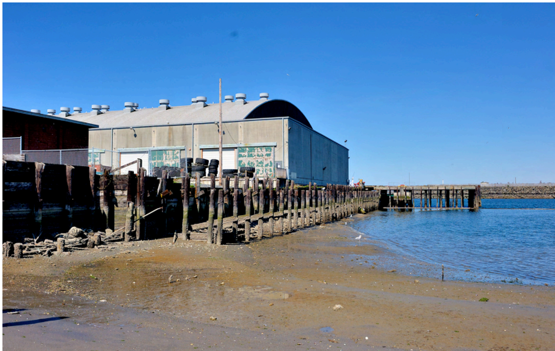
Existing structures along Bellingham Bay
