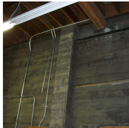
Board Formed Concrete
