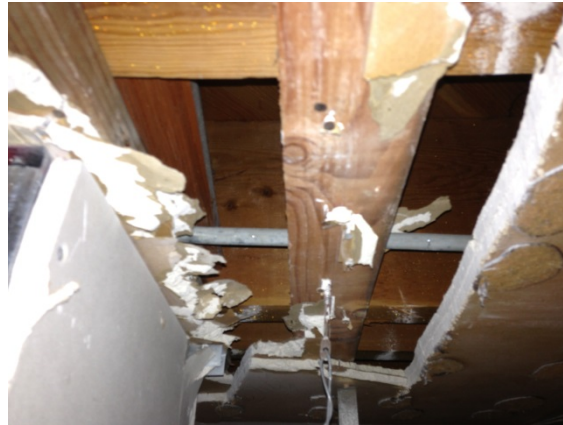
Double Layer of 5/8" GWB at 1 st Floor Clg.
