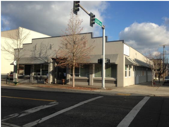
Building to the North
