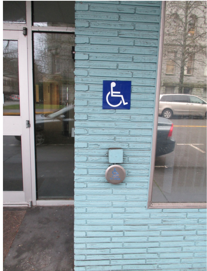
Original Roman Brick – Below many layers of paint
