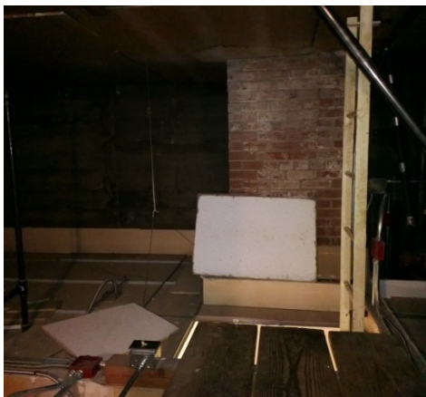
Brick Flue to Roof
