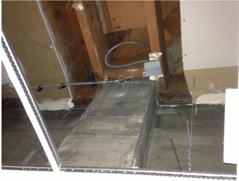
Concrete Pilasters at Exterior Walls
