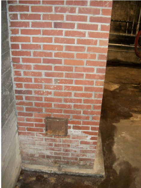
Brick Flue at Sub-Basement
