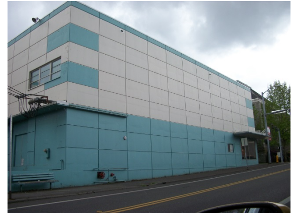
4' x 8' Pattern to Concrete Formwork.
