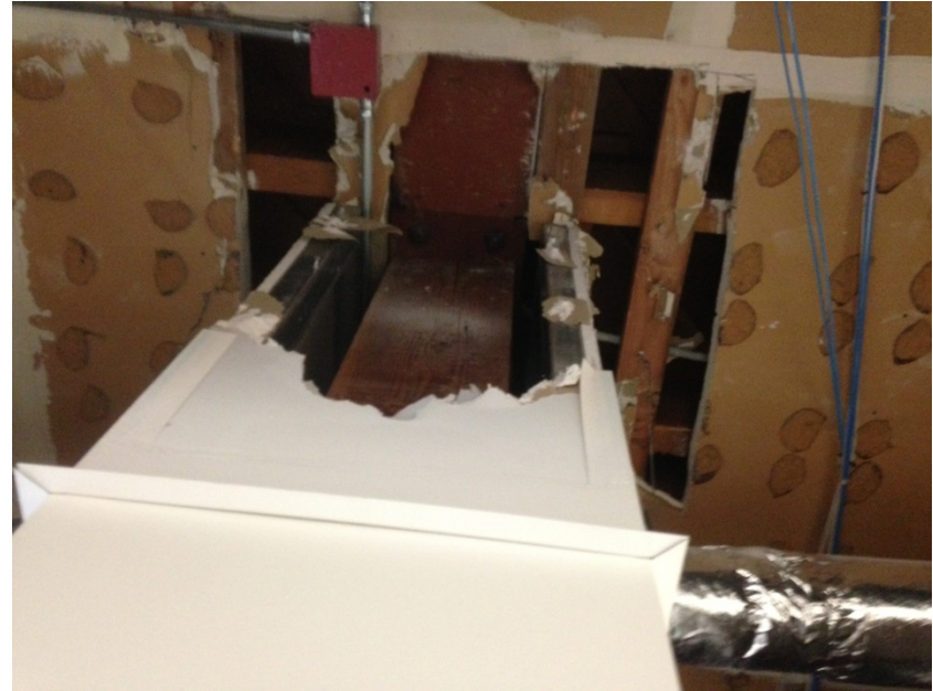
Heavy Timber Columns Supporting Steel Wide Flanges
