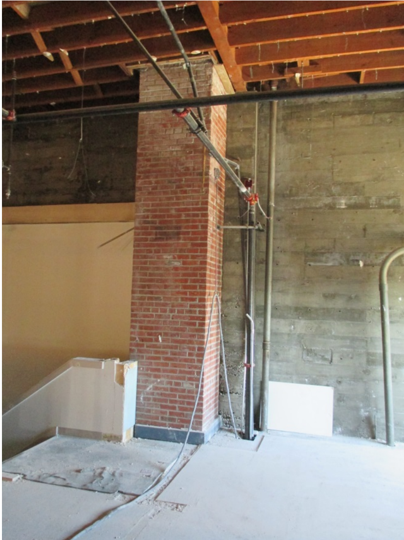
Brick Flue through loft housing level
