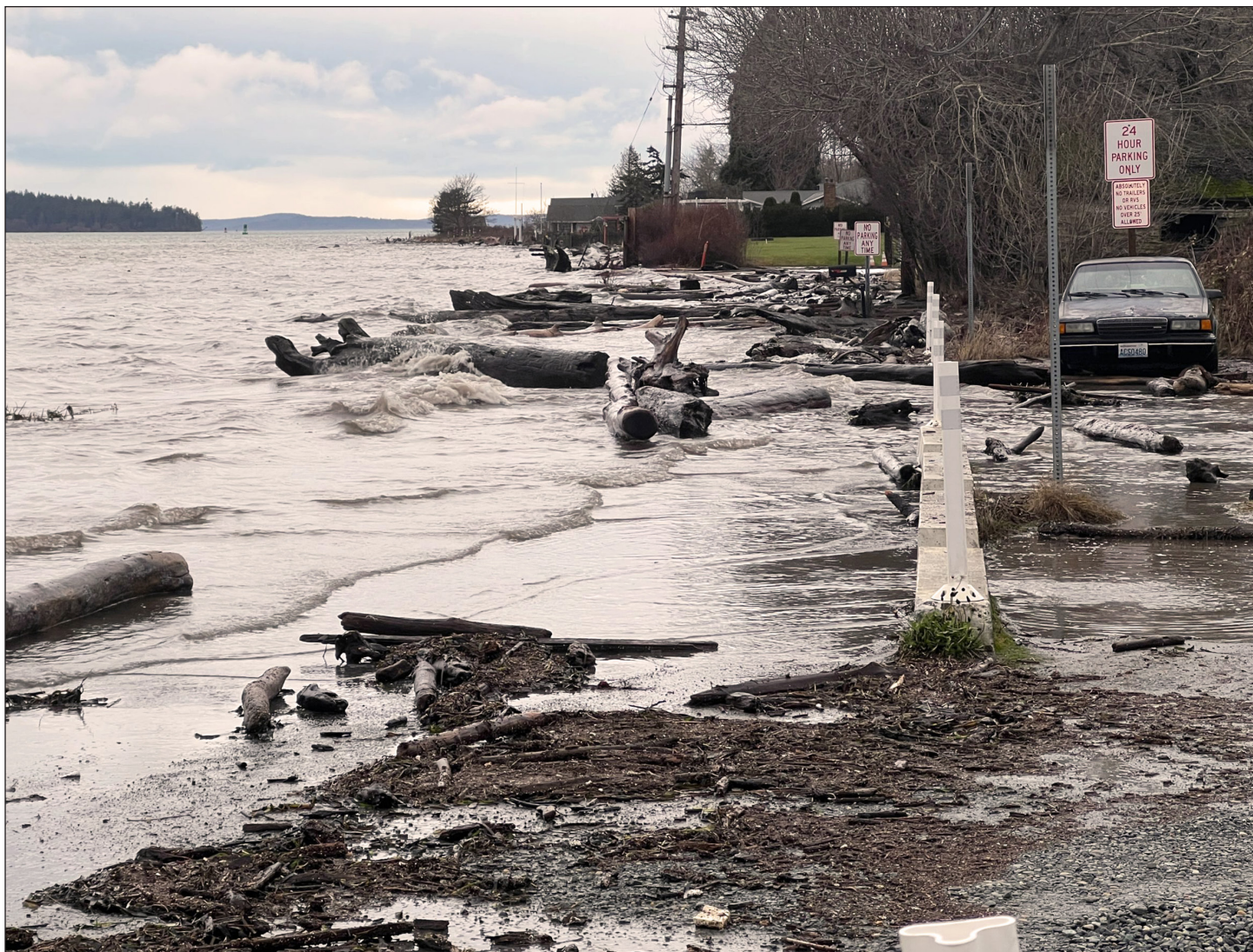
King tide flooding at the Guemes Island ferry lot, 2022. Photo submitted by Sally Peyou to the King Tides program via MyCoast.
